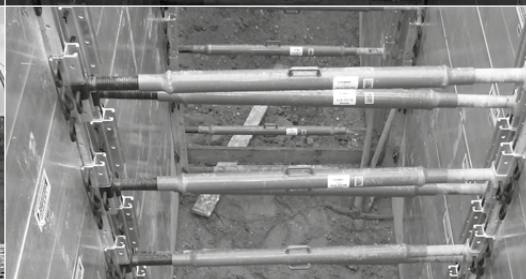
Trench shoring systems
